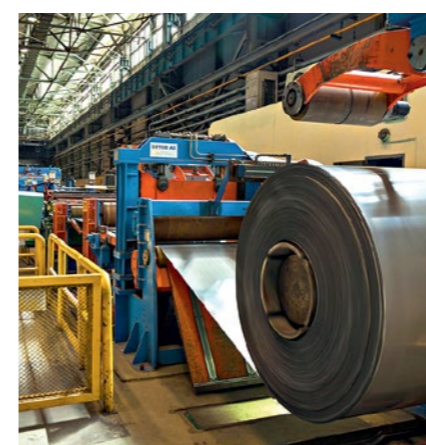
Steel preparation and cutting lines upgrade and construction
