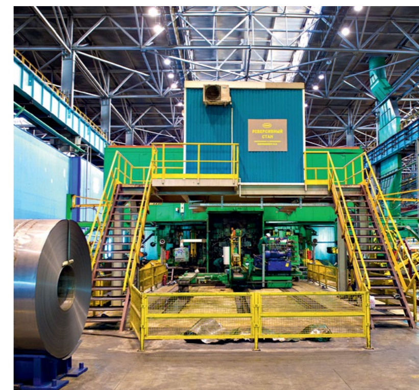
Reversing mill construction
